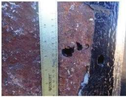
Fig 3 Pitting corrosion and thickness loss in Carnarvon Fascine wall (Carnarvon Fascine Wall Independent Review, K1488, Report R972 Rev 1)
